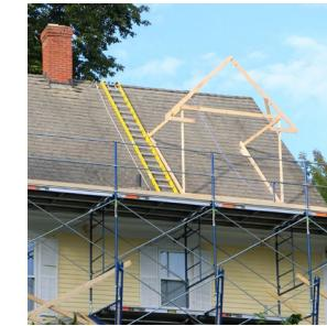
Anchoring and tying the scaffold to a solid structure is essential to prevent tipping or swaying.
