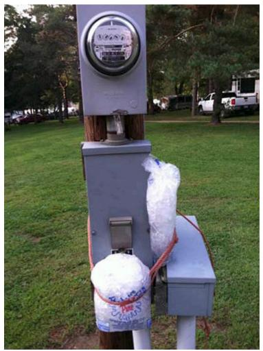
Somebody had the bright idea of strapping on ice bags to cool this electrical panel box after breakers kept tripping. It shouldn't take a physics degree to recognize the dangers of exposing electrical equipment to moisture.
