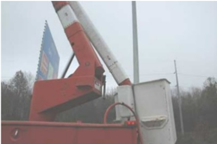
Photo 1: Aerial lift boom after incident. Note that the lower boom section remains elevated while the bucket-end of upper section is in a lowered position (photo courtesy of OSHA).
