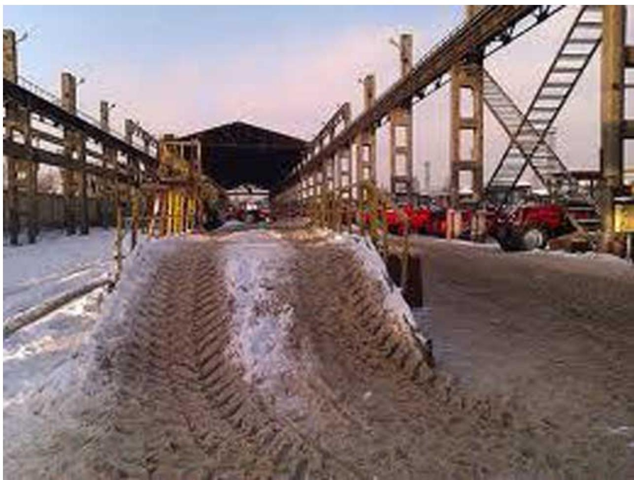
A hazard even in perfect weather conditions, ramps like the one in this picture become an even greater slip-and-fall danger when they're covered in snow and ice. Although it appears that the ramp might have been sanded, it would have been a lot safer had the snow and ice been completely removed.
