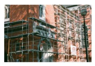
Here's another 'pirate's plank' at a construction site. It appears that while workers can see the windows, they can't always see the light when it comes to ensuring their own safety. One small misstep could have disastrous consequences. Where's the proper scaffolding that is required by law? (WorkSafeVictoria, Australia)
