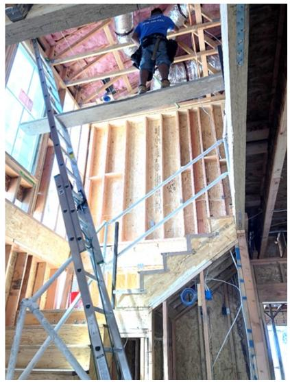
Ingenuity at its finest or accident waiting to happen? The walking space on the plank is limited and awkward which makes any movement dangerous. Reach back for the hammer, lose balance, slam into the stair guardrails on the way to concrete floor below.
