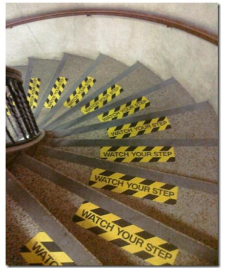
A "watch your step" sign at the top of a stairway is a good safety reminder, but this photograph illustrates too much of a good thing. Every step on this stairway has a safety warning, which could actually end up distracting a worker and causing a serious fall. (www.safetyrisk.net)
