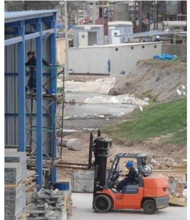
It's a bit hard to make out, but the workers in this picture are using the forks of the forklift to support one end of the scaffolding another worker is working on. This is an unstable and dangerous arrangement that violates OSHA requirements for supporting scaffolds (Sec. 1910.28(a)(2) for General Industry, Sec. 1926.451(c)(2)(v) for Construction).
