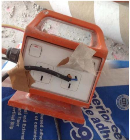
Making do with what you have is good advice in many situations, but in the world of workplace safety, making do often translates into taking unsafe shortcuts. Here we have a situation where someone has shoved bare electrical wires into an electrical outlet and then taped the makeshift wiring to hold it in place. Hopefully necessity won't become the mother of electrocution. (WorkSafeVictoria, Australia)
