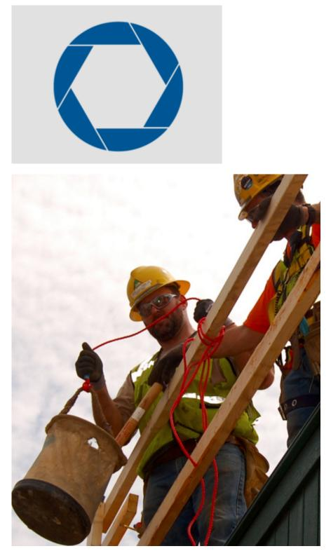
Picture This nearly always focuses on unsafe work practices, but this week we have a photograph showing workers doing the right thing. In this case, a worker is shown using a bucket and rope to hoist tools to an elevated work area. This arrangement allows workers to maintain three points of contact when ascending or descending ladders. (eLCOSH)
