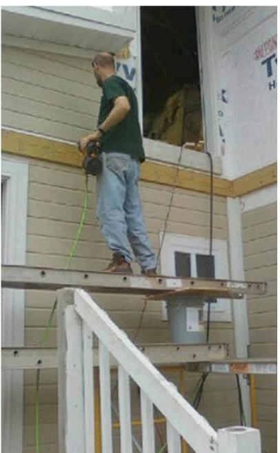
The ladder arrangement—metal ladders stacked on a bucket—in this photo would actually be considered a "scaffold," i.e., a temporary elevated platform and supporting structure used to support workers, by OSHA (under Sec. 1910.21(f)(27)). And according
