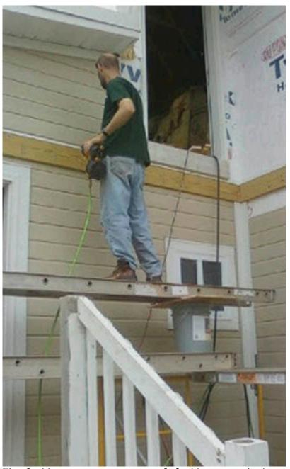
The ladder arrangement—metal ladders stacked on a bucket—in this photo would actually be considered a "scaffold," i.e., a temporary elevated platform and supporting structure used to support workers, by OSHA (under Sec. 1910.21(f)(27)). And according to OSHA rules (Sec. 1910.28(a)(2)), scaffold footing or anchorage must be "sound,
