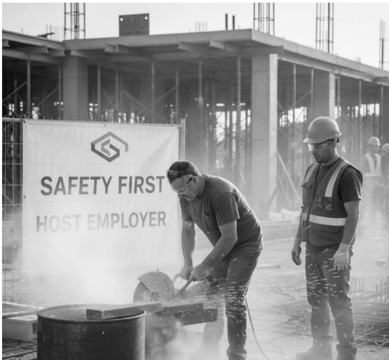
In the image, the contractor is cutting metal with a powered saw while producing heavy sparks and dust, yet he still lacks the required PPE—no face shield, no hearing protection, and no respiratory protection. He is working inches away from another subcontractor who also has inadequate PPE and is standing directly in the spark path. Despite the large "SAFETY FIRST – HOST EMPLOYER" sign behind them, neither worker is
