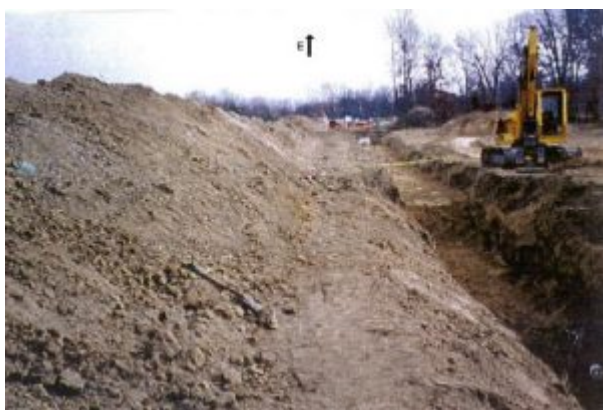
Sewer Installation Project (Trench pictured is approximately 200 feet long.)
