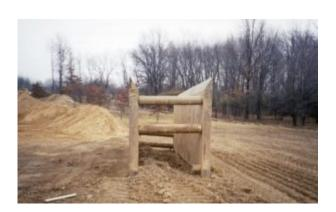
Figure 2. Shield (Shield was removed from the trench with an excavator and placed 20 yards from the trench.)
