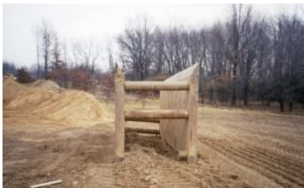
Figure 2. Shield (Shield was removed from the trench)
