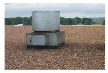
Exhaust fan had been removed for cleaning, creating a temporary opening where cleaner fell approximately 35 feet/10 meters onto a piece of machinery in the factory.
